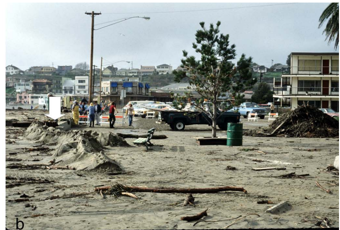
Figure 6. (a) Overtopping of low seawall at times of elevated sea levels and large waves has repeatedly flooded the esplanade area of Capitola, with significant damage to commercial development. (b) Sand and debris deposited when waves overtopped the low seawall along Capitola's esplanade. View similar to (a). Arrow points to the same seawall in (a).
