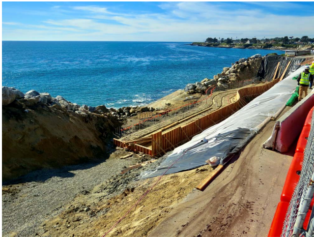
Figure 20. Excavation and site preparation for seawall construction along West Cliff Drive in Santa Cruz after January wave damage (November 2023).
