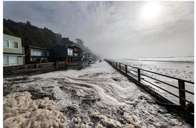
Figure 24. Waves at high tide on 28 December 2023 overtopped the seawall and again flooded Beach Drive (photo credit: Kevin Painchaud, Lookout Santa Cruz).
