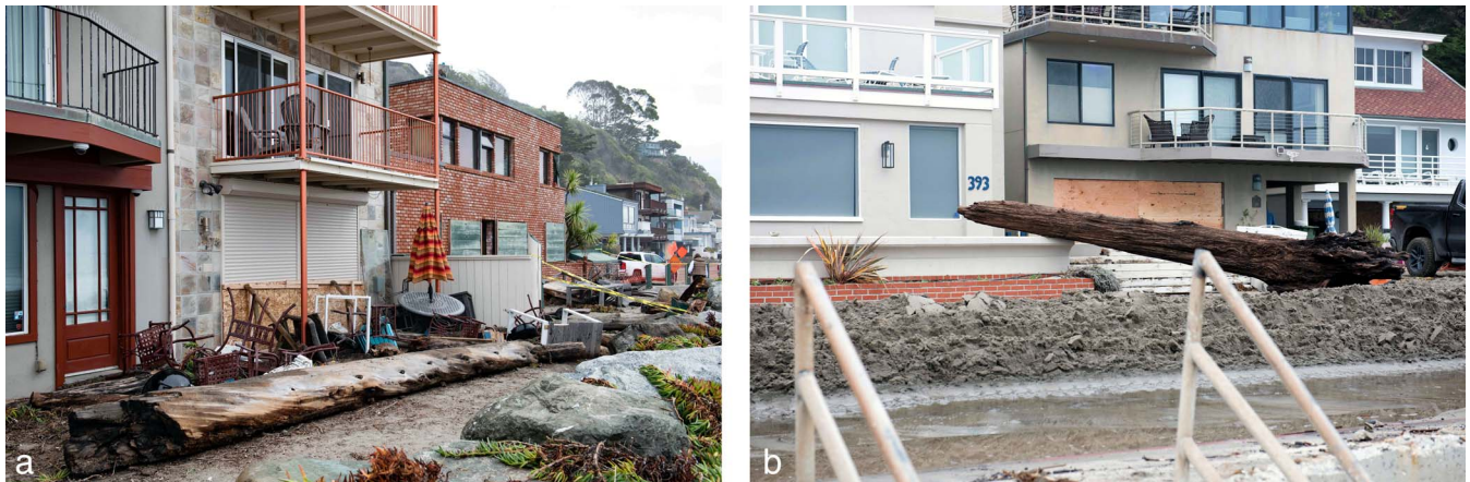
Figure 18. (a) Logs and debris were carried over the low rock revetment and deposited on patios of homes along Beach Drive in Rio del Mar. (b) Beach sand and logs were carried over the low seawall, threatening back beach homes (photo credit: Kim Steinhardt).
