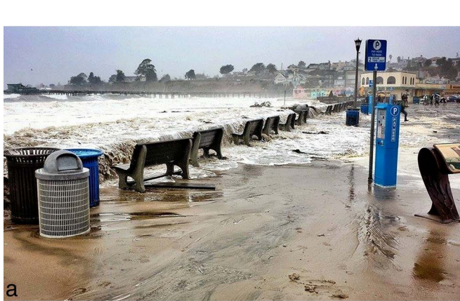
Figure 6. (a) Overtopping of low seawall at times of elevated sea levels and large waves has repeatedly flooded the esplanade area of Capitola, with significant damage to commercial development. (b) Sand and debris deposited when waves overtopped the low seawall along Capitola's esplanade. View similar to (a). Arrow points to the same seawall in (a).
