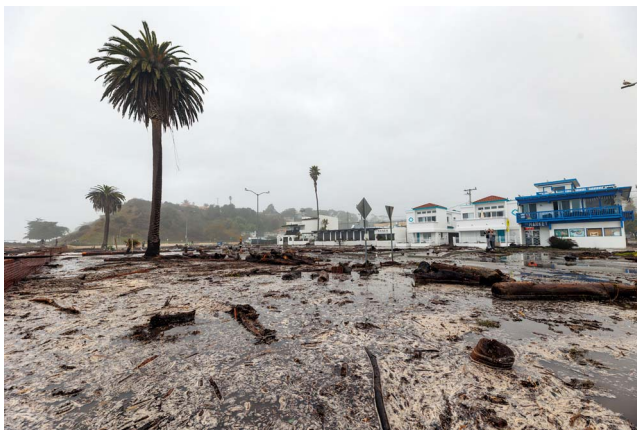
Figure 23. Large wave at high tides in late December 2023 washed over the seawall and onto the esplanade, leaving logs, sand, and debris in the parking area (photo credit: Kevin Painchaud, Lookout Santa Cruz).
