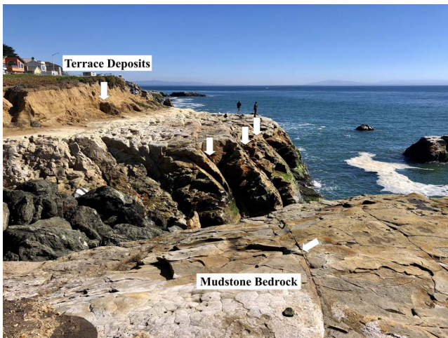
Figure 11. Typical section of coastal bluff along West Cliff Drive with pervasively jointed mudstone bedrock capped by terrace deposits. Slab failure typically occurs along the steeply dipping joint sets (arrows) that produce a ramp allowing large waves to overtop the bedrock and erode the overlying highly erodible terrace deposits.
